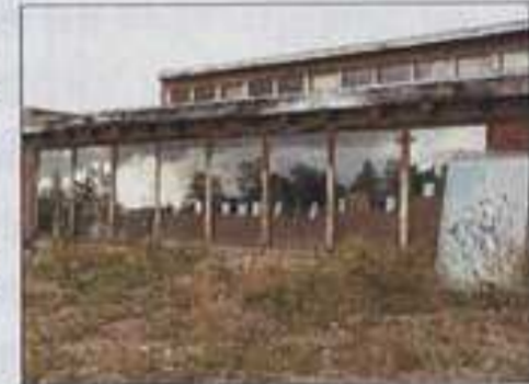
Joseph's house—side view
