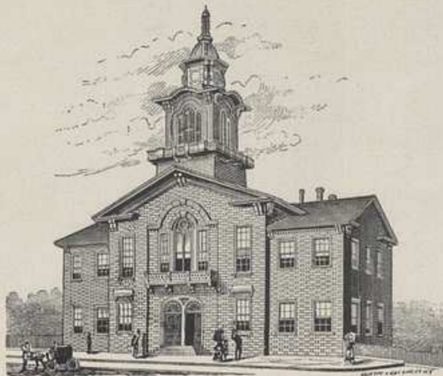
COURT-HOUSE, LEHIGH COUNTY, ALLENTOWN.
