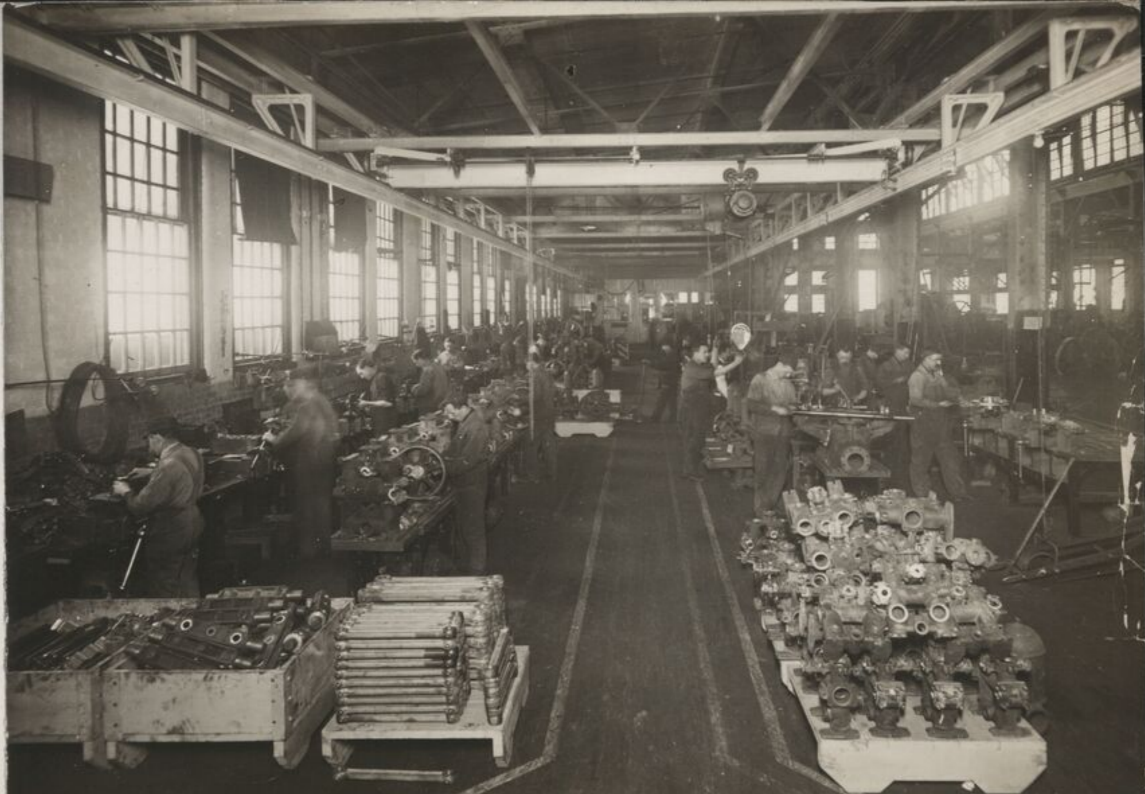
ASSEMBLING SMALL POWER PUMPS, POWER PUMP PLANT
