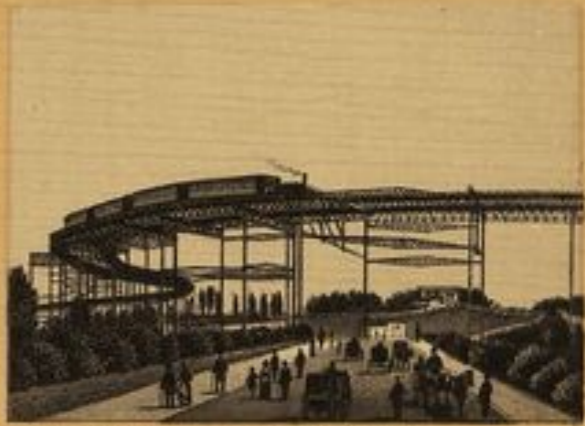
HIGH CURVE ELEVATED RAILROAD W 110TH STREET
