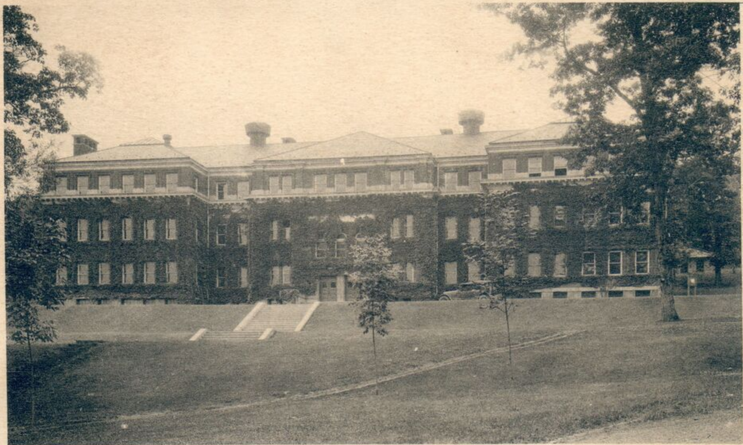
WILLIAMS HALL, MECHANICAL ENGINEERING—LEHIGH UNIVERSITY. BETHLEHEM, PA.
