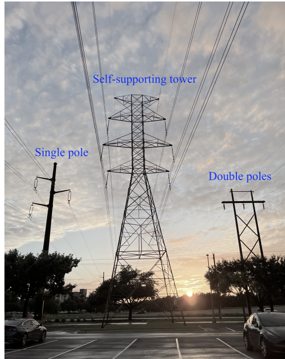
Figure 3.4: Examples of transmission line supporting structures: a single pole, a self-supporting tower, and a double pole.
