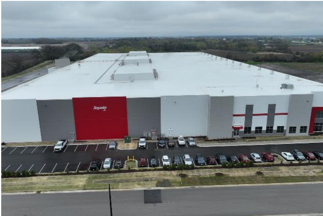
Figure 2 Commercial TPO application: Saputo Cheese USA Facility in Caledonia, Wisconsin
