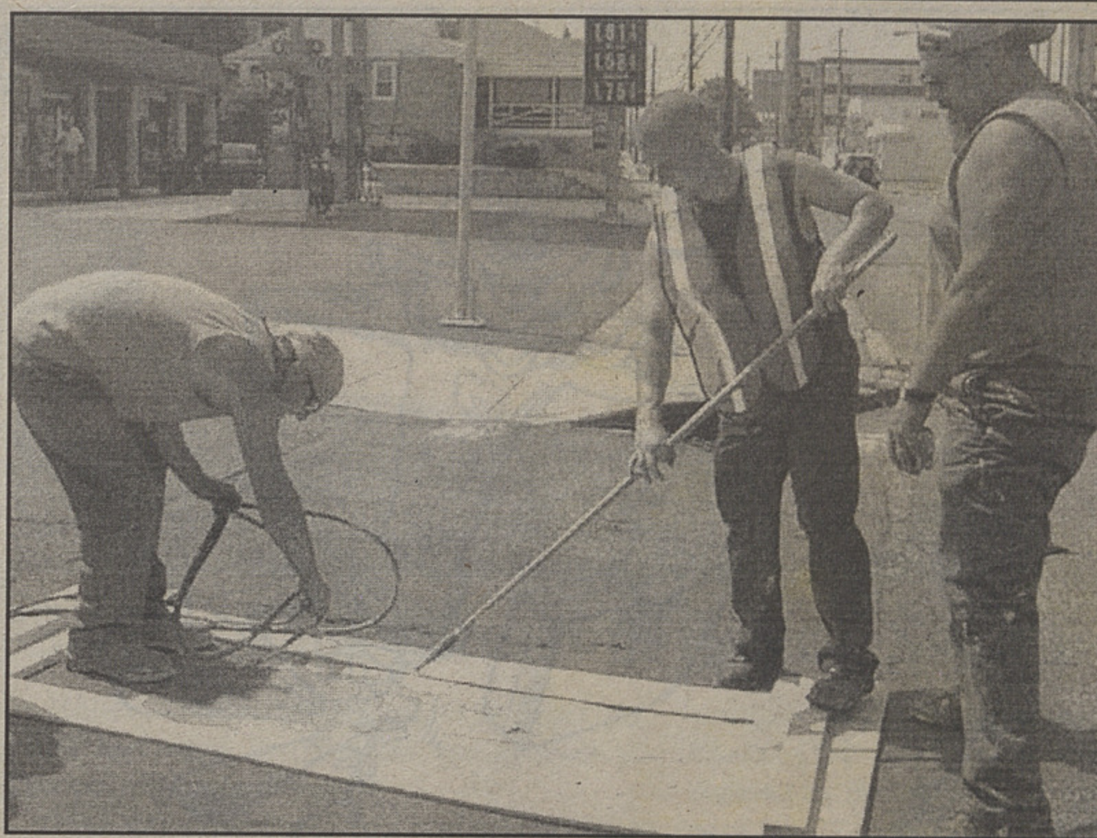
Hellertown workers Lance Eure, Joe Luybli and Bruce Yonney paint the crosswalk at Linden and Main streets. The new design paint job will help make Hellertown's streets, especially Main Street, more pedestrian friendly.
