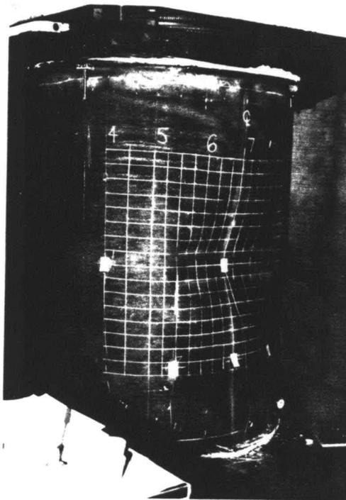
**Figure 2:** Axial Test on 60-inch Diameter Specimen
